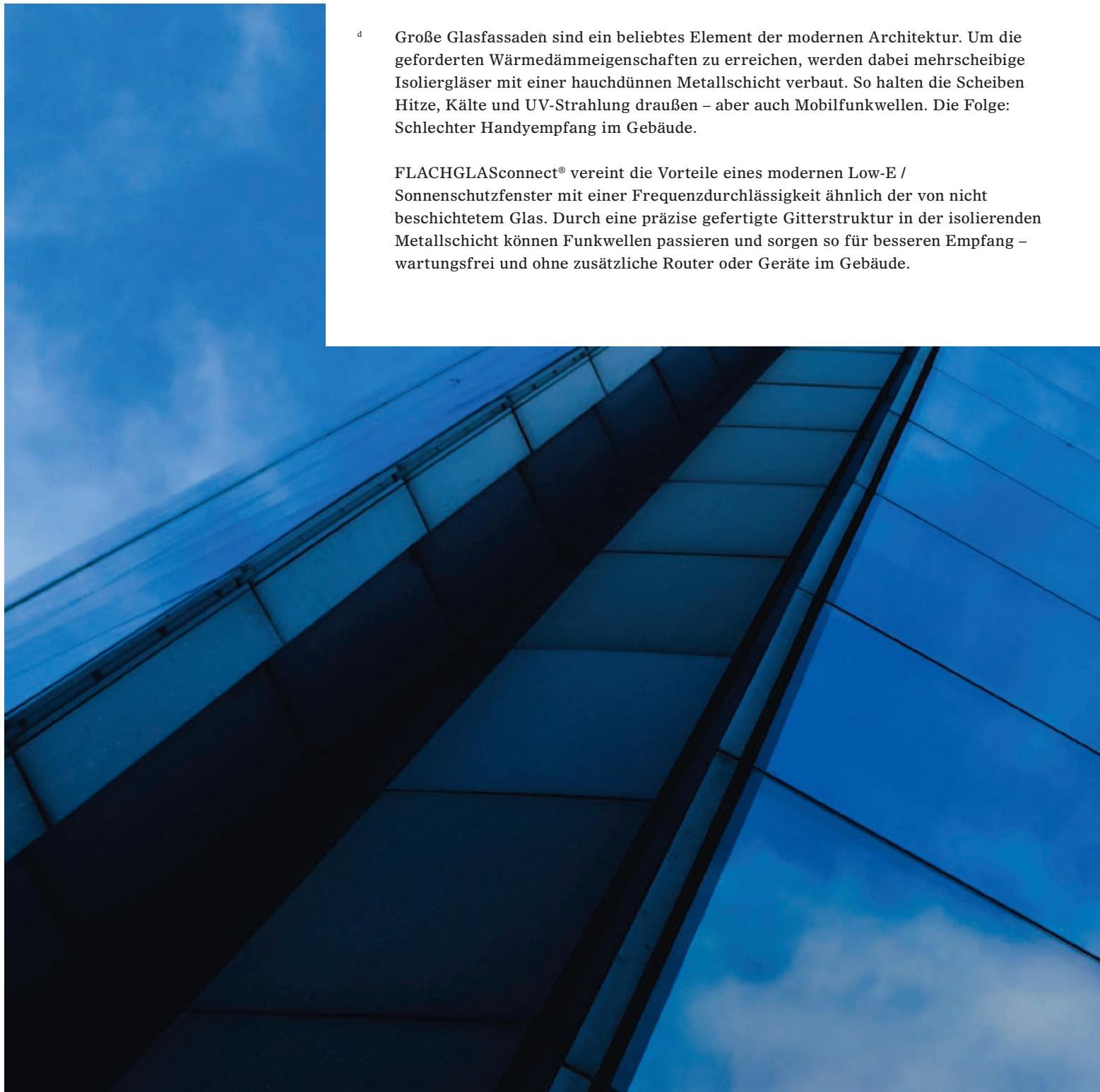
Large glass façades are a popular element of modern architecture. To achieve the required thermal insulation properties, multi-layer insulated glazing units are installed with an extremely thin metal coating. This means that the windows keep the heat, cold and UV rays outside – but also mobile phone waves, resulting in poorer phone reception inside the building.
